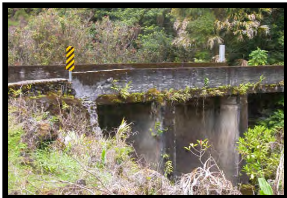
Mokulehua (mm 28-29, built 1908) Showing 48 foot concrete slab deck supported by two piers with a solid slab railing. Oldest bridge in East Maui.
